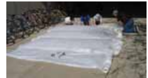
Figure 8: Polyethylene being rolled up to hoist into place.
