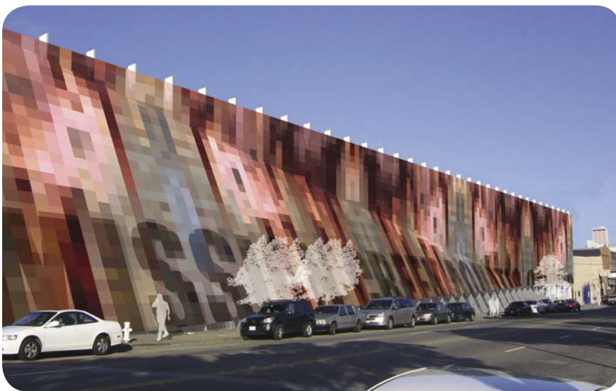
Figure 1: The billboard facade along Folsom Street.
